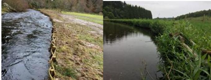
Photo 2: Willow spilling on the River Avon (left: immediately after, right: 2 years after installation)
